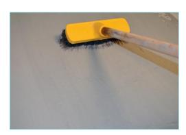
Crystalline waterproofing material consisting of emulsion polymer based liquid and cement based powder components that contain chemical additives to increase water impermeability and workability, which is applicable from both negative and positive directions of interior and exterior concrete and masonry structural
